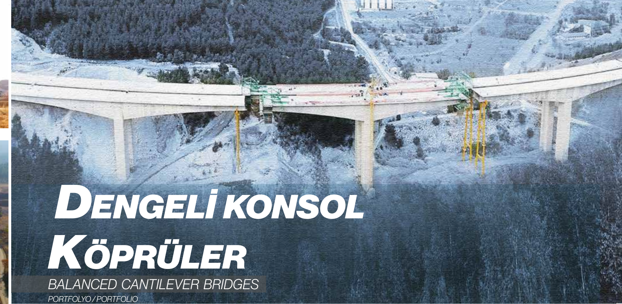
ŞEHZADELER VİYADÜĞÜ | AMASYA/TÜRKİYE Dengeli Konsol (BCM) / Ardgerme Metodu ŞEHZADELER VIADUCT | AMASYA/TURKEY Balanced Cantilever / Post-tensioning Method
