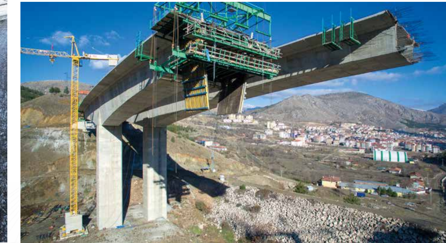
ŞEHZADELER VİYADÜĞÜ | AMASYA/TÜRKİYE Dengeli Konsol (BCM) / Ardgerme Metodu ŞEHZADELER VIADUCT | AMASYA/TURKEY Balanced Cantilever / Post-tensioning Method
