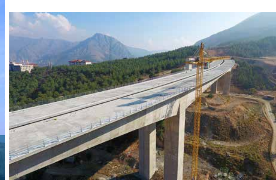
İMRAHOR VİYADÜĞÜ | ANKARA/TÜRKİYE Dengeli Konsol (BCM) / Ardgerme Metodu İMRAHOR VIADUCT | ANKARA/TURKEY Balanced Cantilever / Post-tensioning Method
